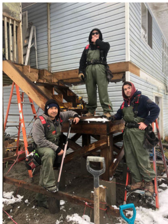
Students replacing stairs with a landing
