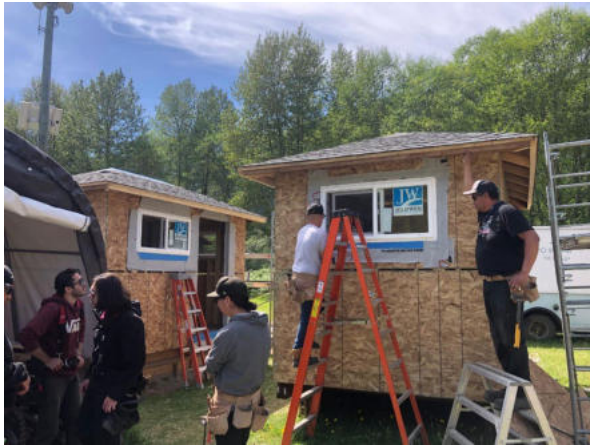
Students installing windows and doors
