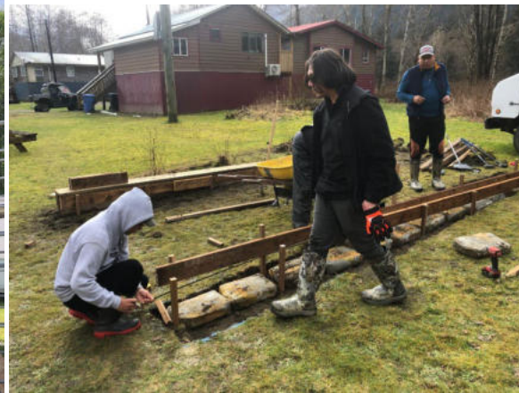
Students preparing a level foundation for sheds
