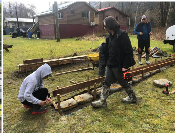
Students preparing a level foundation for sheds
