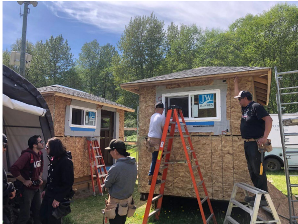
Students installing windows and doors
