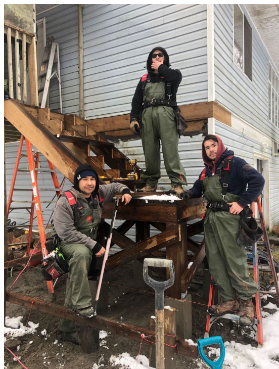
Students replacing stairs with a landing
